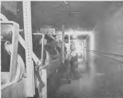
ARUBA'S ONLY tunnel stretches 50 feet underground below the storage piles in the picture above. The machinery at left controls the flow of materials from storage to use via conveyor.
